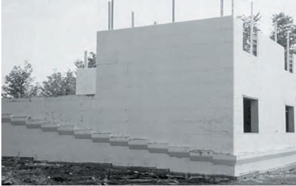
The various form units have cores of 4" (102mm), 6" (152mm), 8" (203mm), 10" (254mm) and 12" (305mm), with an overall thickness of 9 1/4" (235mm), 11 1/4" (286mm), 13 1/4" (337mm), 15 1/4" (387mm) and 17 1/4" (438mm) respectively. The BLE can be used at any elevation on the wall on either side. The form is 32" (813mm) long x 13 1/2" (343mm) deep.
